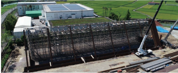
④両側斜壁面鋼矢板構築
