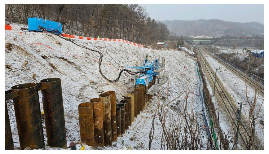
The GYRO PILER™ is installing piles in a emergency disaster recovery work (Retaining wall is being constructed along the railroad track for slope failure measure.)
