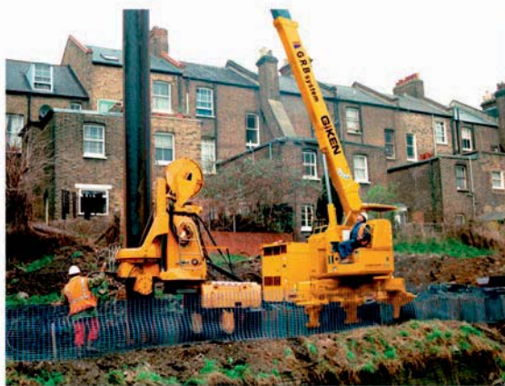
◀ Overseas construction site (London)
