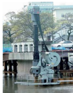
Sheet piling on the water
