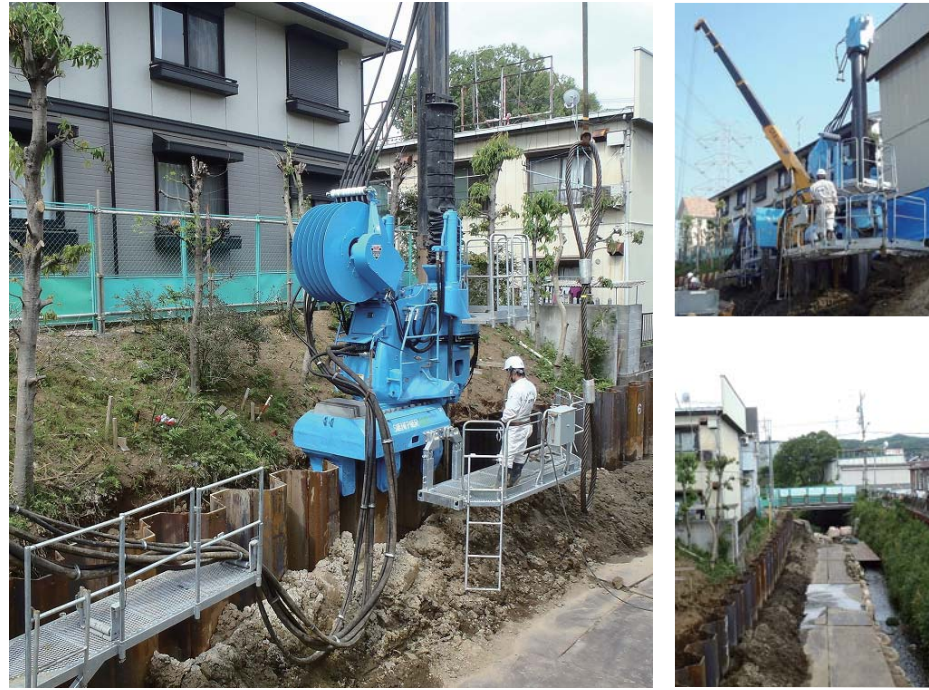
Project : Machida City Public Sewer System, Storm-Water Sewer Construction Works Location : Machida City, Tokyo Period : May 2013 Silent Piler : F201 Type of Sheet Pile : U Sheet Pile SP VL Pile Length : 27.89 ft
