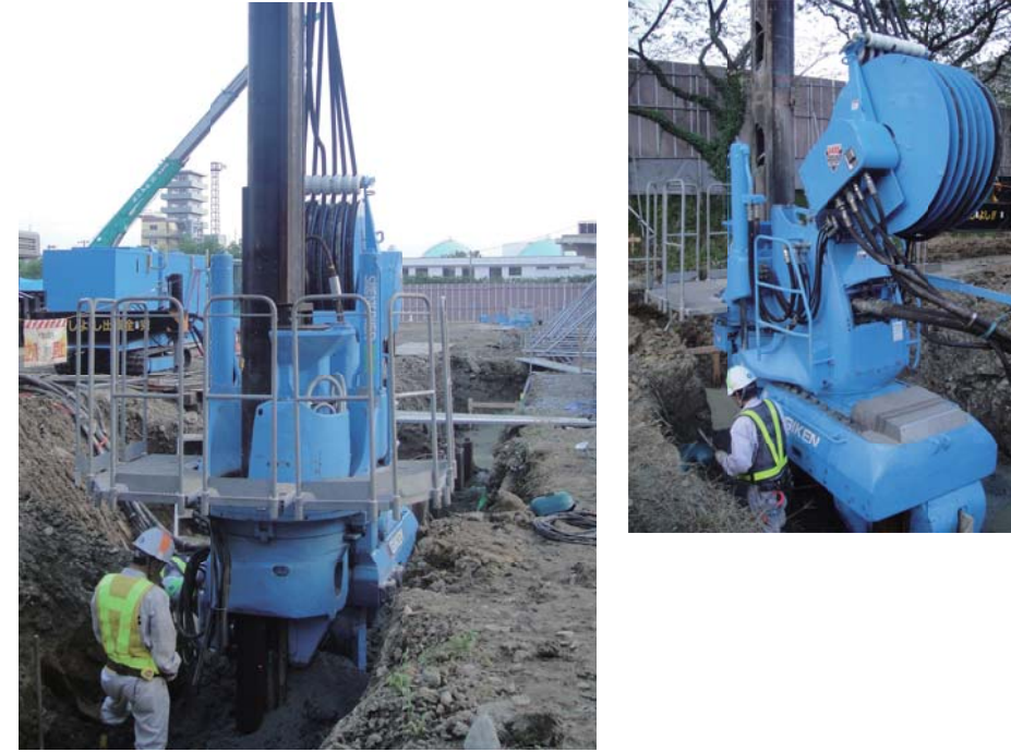
Project : Demolition of Miyagi Prefectural Public Health and Environment Bldg.- Second Phase Location : Sendai City, Miyagi Period : October 2013 ~ November 2013 Silent Piler : F201 Type of Sheet Pile : J Pocket Pile JFESP-4WS, U Sheet Pile SP IIw Pile Length : 13.12 ~ 24.61 ft
