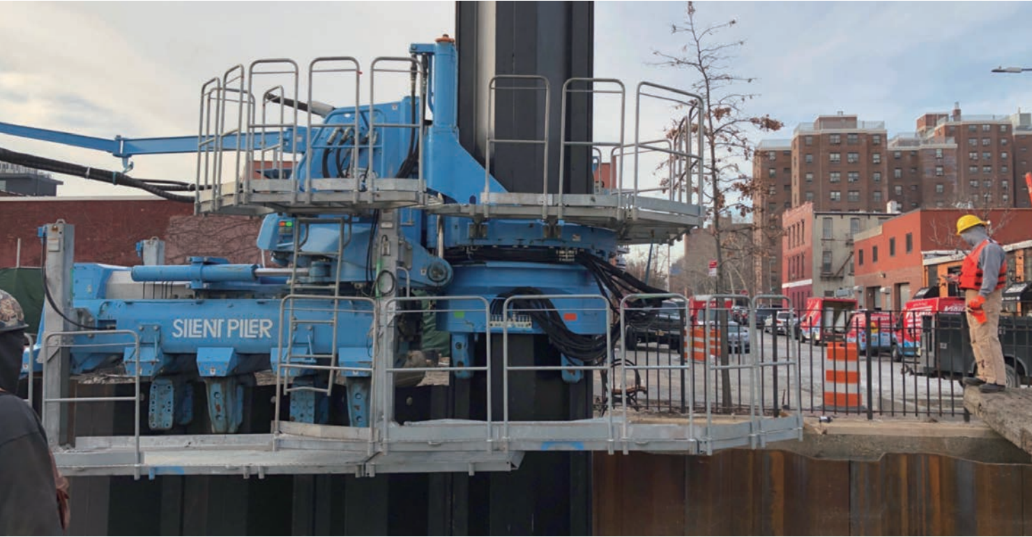
Installing the last sheet of the alignment next to the adjacent section
