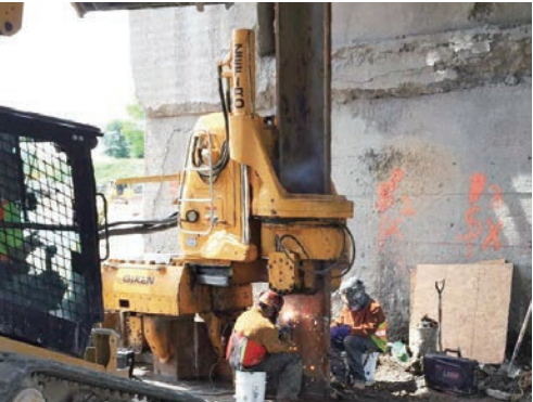
Spliced Pile Welding
