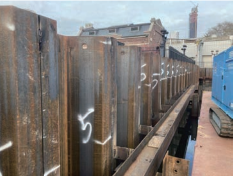
Falsework to support the sheets
