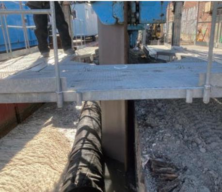
Sheet piling in front of existing bulkhead
