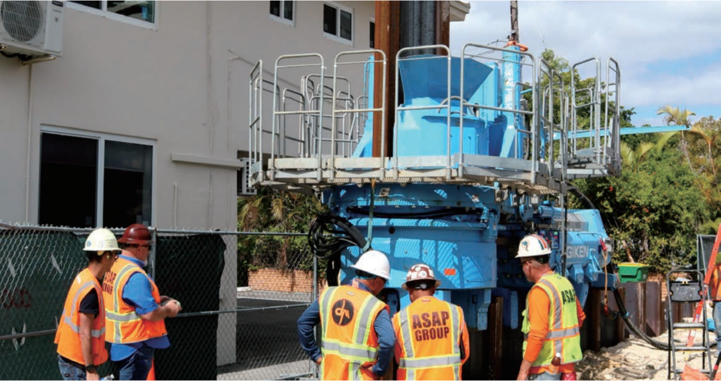
Vibration free machine to install sheet pile by radio control
