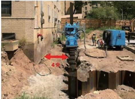
Piling Adjacent to Existing Structure
