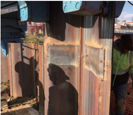
Welded Splice Plates
