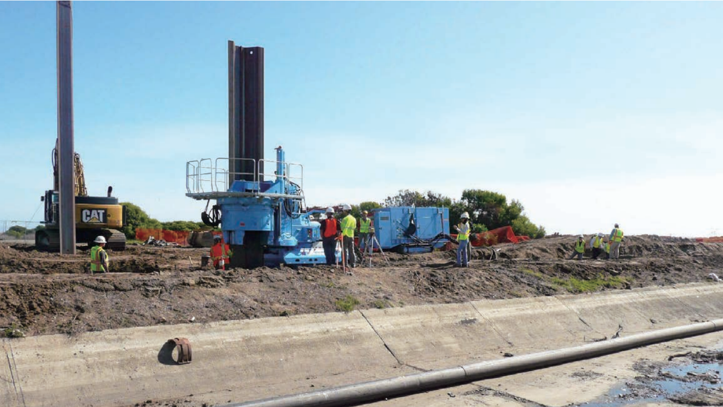
Sheet Pile Installation
