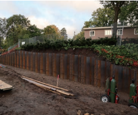
Sheet Piles After Installation
