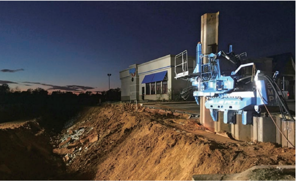
Top: After Parking Lot Collapse Bottom: Sheet Piling
