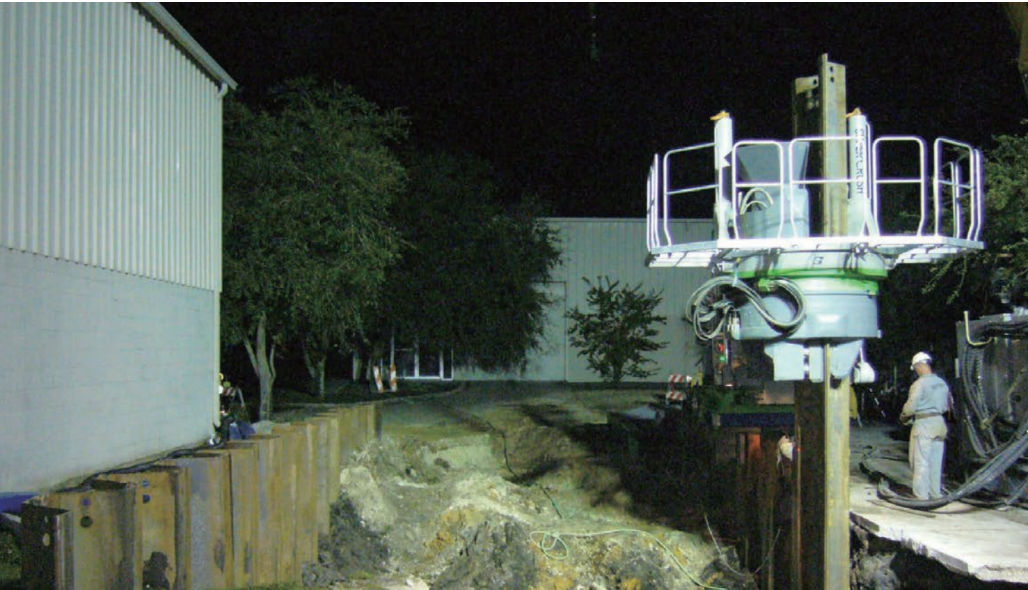
Sheet Pile Installation
