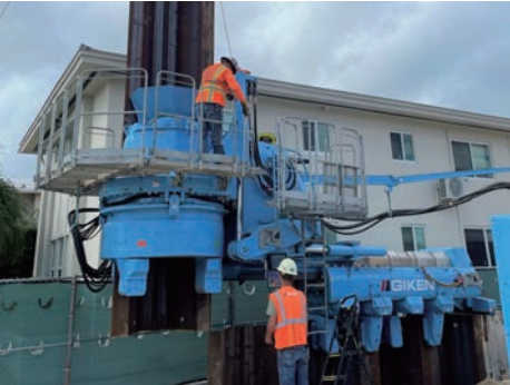
PILER STAGE™ for pitching sheet pile safely
