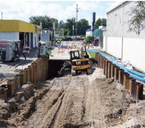
Completion of Sheet Piling
