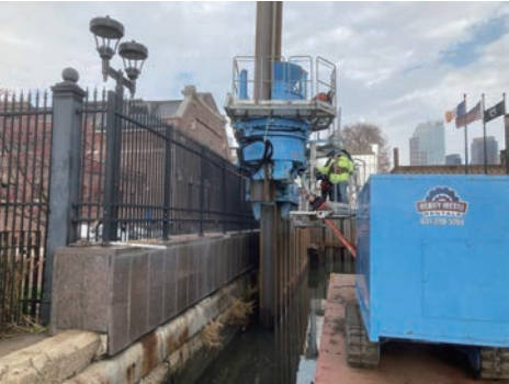
Sheet piles in front of existing wall
