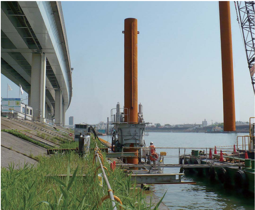
Using the Tubular Sheet Pile Press-in Method to build an urban river revetment close to a motorway
