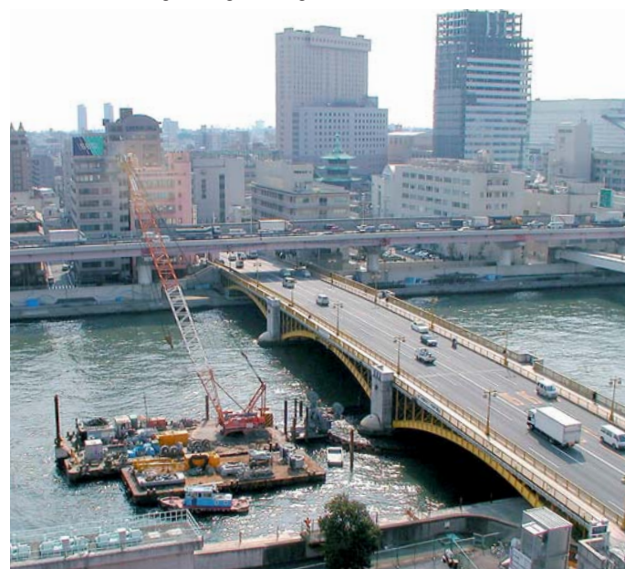
Antiseismic Strengthening of Bridge Pillars
