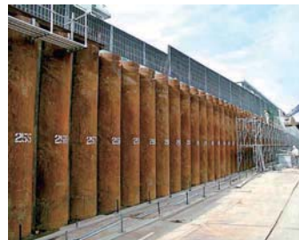
The Giken Wall as seen after excavation work.
