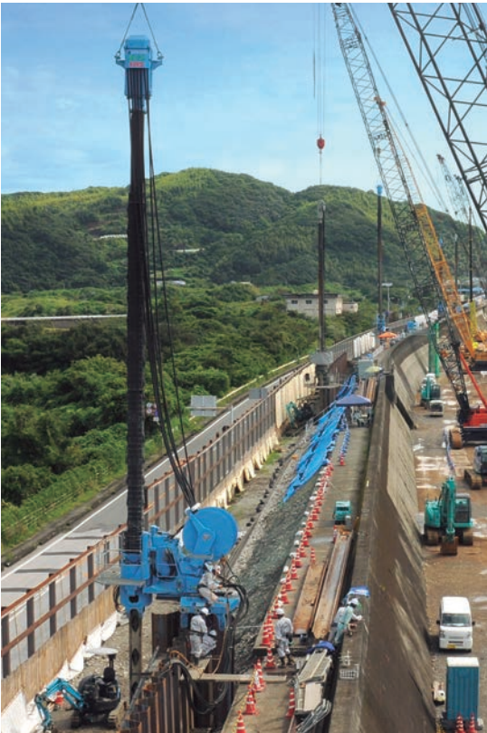
Liquifaction Prevention Works for Reinforcing Seacoast Levee with Double Sheet Pile Cut-off Wall Kochi, Japan
