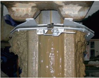
(1) Fitting Casing Scraper around the Casing.
