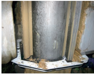
(2) Fixing the Casing Scraper with catch clip.
