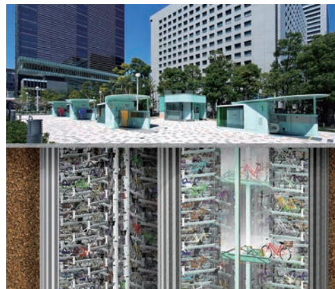
Earthquake-resistant underground bicycle parking ECO Cycle (Minato-ku, Tokyo)
