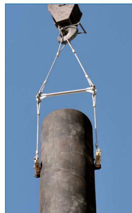
The Spreader Beam can prevent kink, wear or damage on sling wire ropes. It makes pitching work safer and more efficient. The lightweight and compact spreader beam can be used for 2 to 4 different diameter piles.
