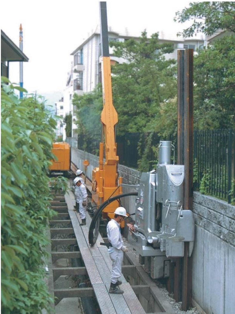
Building a Wastewater Structure in a Narrow Site with the Zero Clearance Method
