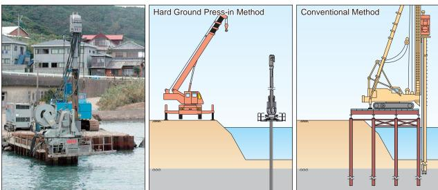
Adjacent to Structure: There is no working time restriction, because it is such a safe method that there is no risk of the machine overturning.
