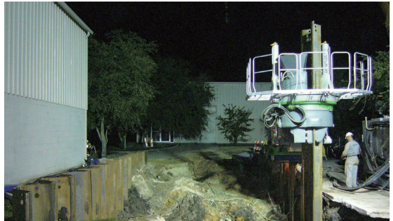
Sheet Pile Installation
