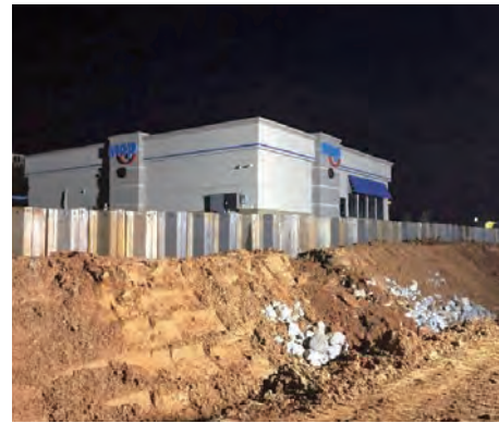
Completion of Sheet Piling
