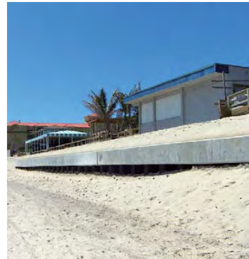
New Seawall (After Completion)
