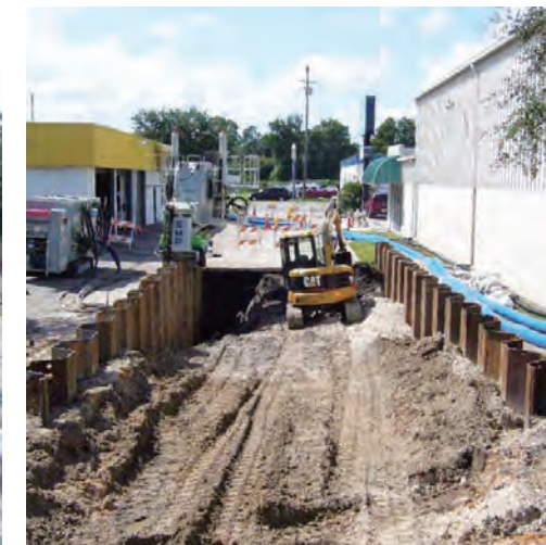
Completion of Sheet Piling
