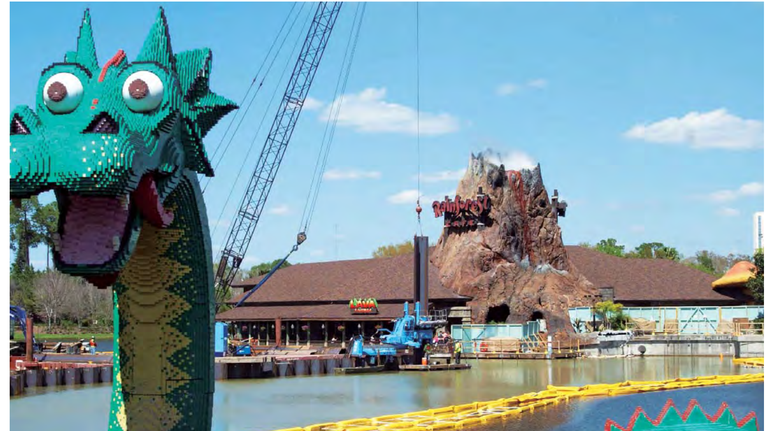
Sheet Pile Installation
