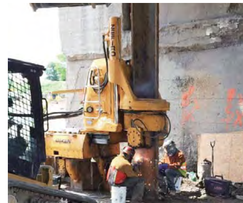
Spliced Pile Welding
