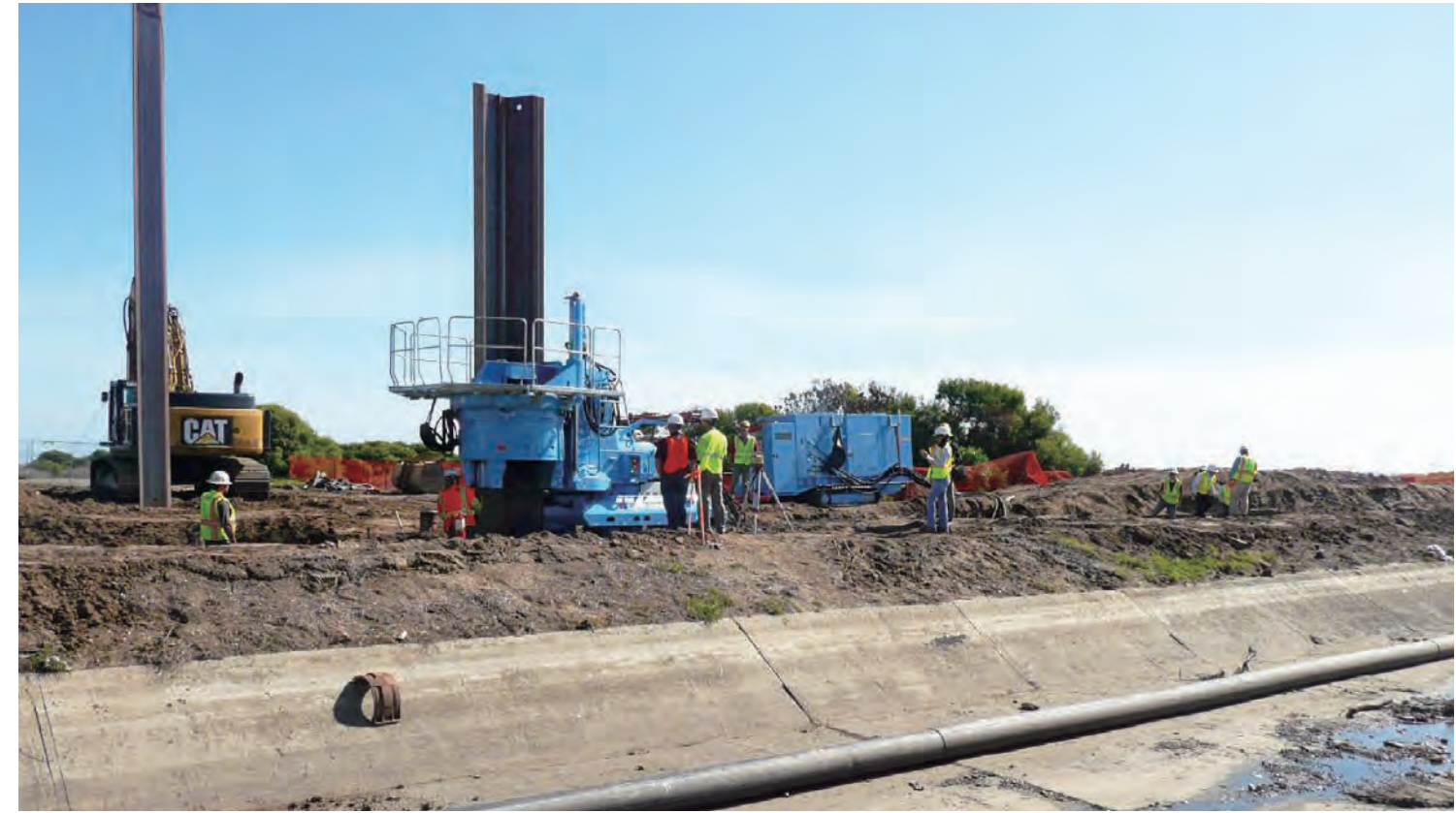
Sheet Pile Installation
