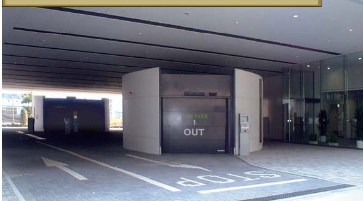
Pilotis (Entrance booths : Car Park 1 (foreground) and Car Park 2 (background))
