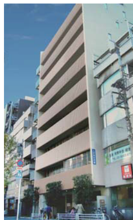
Complete View of Complex Building
