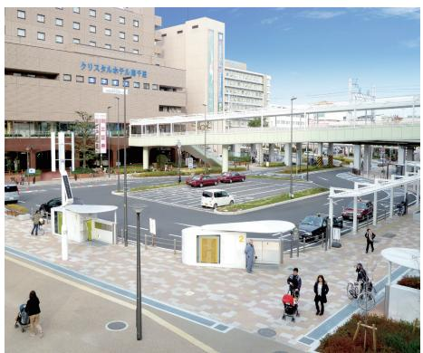
As public bicycle parking lot in Kansai Region, an underground mechanical parking lot was installed for the first time. Along with the station-front redevelopment project of the Hankyu Railway Minamisenri Station, 2 ECO Cycle units were built at the traffic circle. By concentrating several aboveground bicycle parking lots to the underground of the train station plaza, the space in front of the station is utilised effectively and highly convenient parking has become available.
