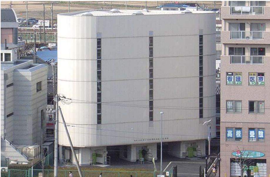
This aboveground bicycle parking lot has a steel frame structure and can hold up to 720 bicycles. It was built in a narrow plot of about 430 m<sup>2</sup> alongside the Sotetsu railway line near Ebina Station. The efficient layout of 4 Eco Cycle units plus an administration block ensures smooth user traffic flows.
