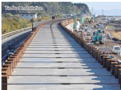
Figure 11: Application of Twin Sheet Pile Walls
