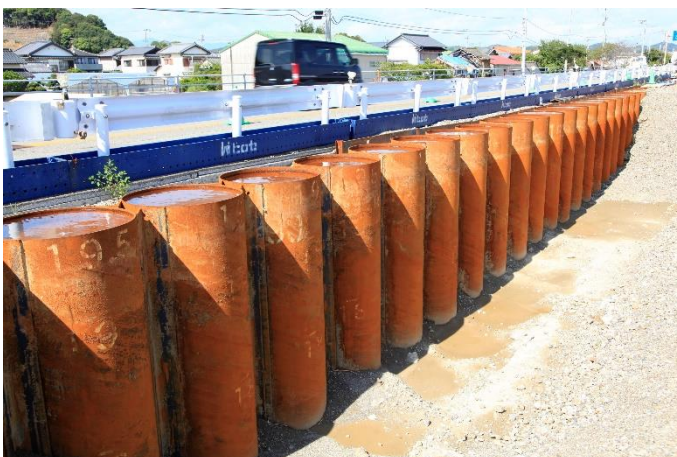
Figure 12: Application of Tubular Pile Wall
