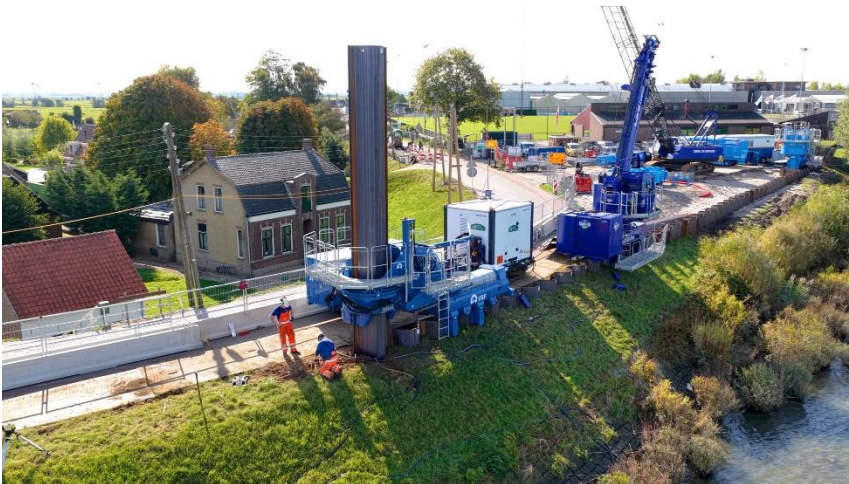
Press-in construction for the Delta Programme (KIJK project)
