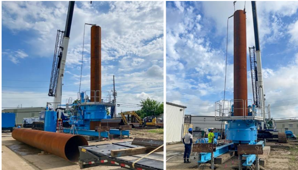
GYRO PILER installed in the United States
