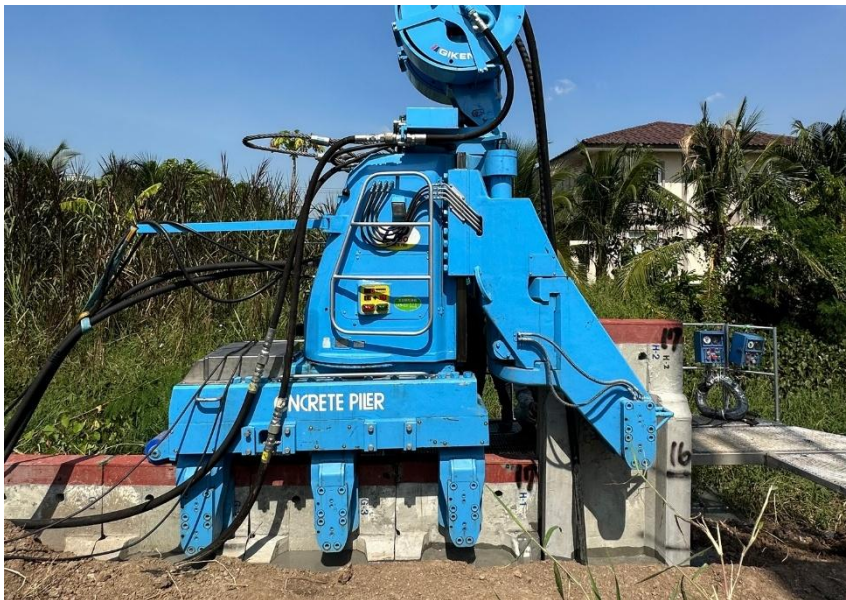
Scene of trial installation of concrete sheet piles
