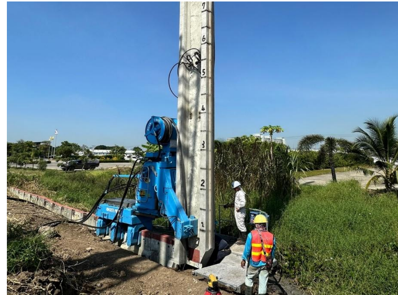
Scene of trial installation of concrete sheet piles
