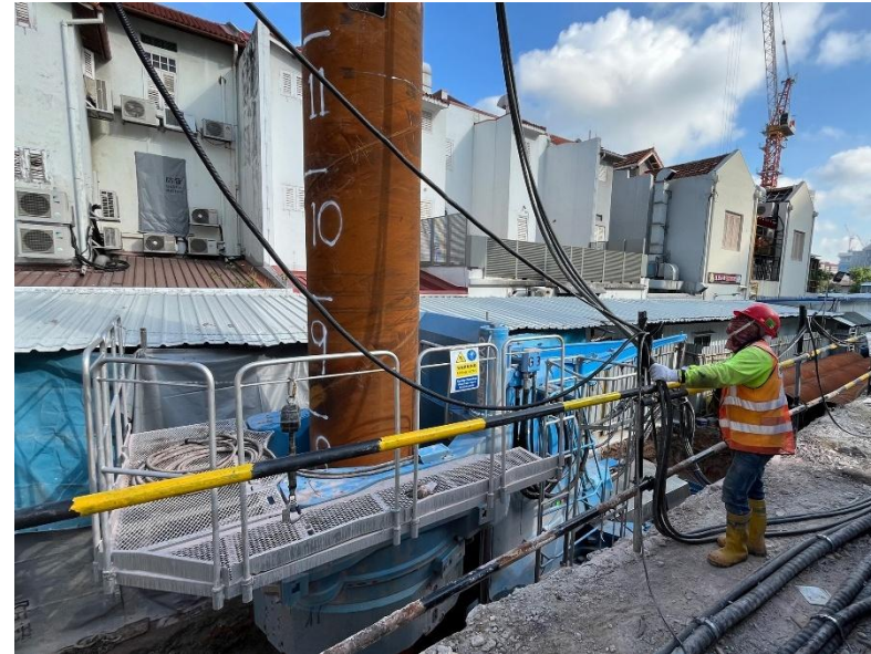
Earth-retaining work for a hotel project adopting the Gyropress Method
