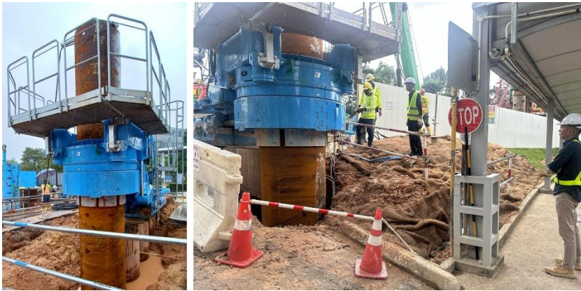
Site adopting Gyropress Method in Singapore
