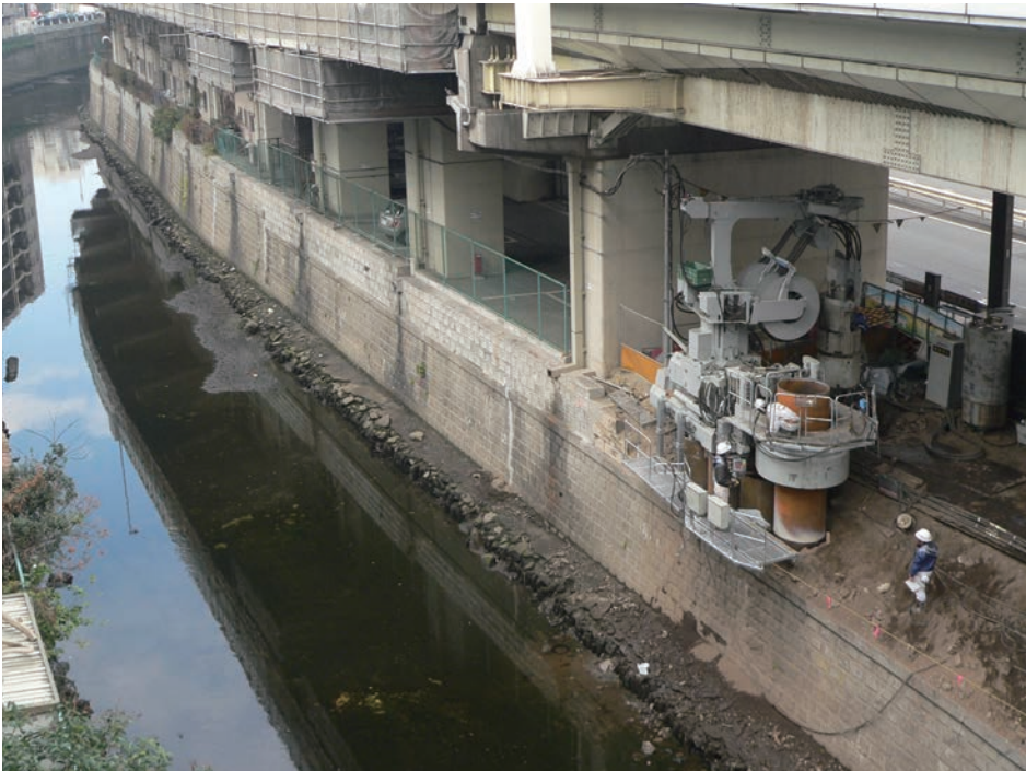
River Bank Reinforcement in central urban area by Gyropress Method
