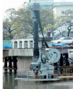
Sheet piling on the water
